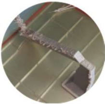
Poor adhesion
